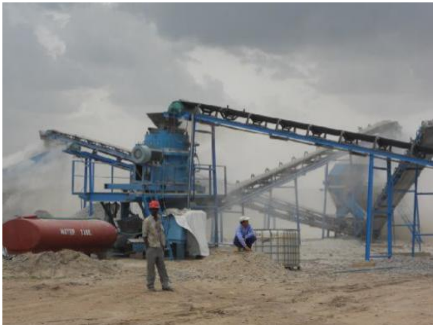
150-200t/h granite crushing plant in Nigeria-2
