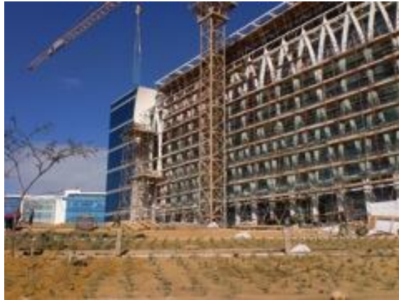
Figure II-3 Construction of Dar Al-Handasa New premises, smart village, Giza, Egypt
