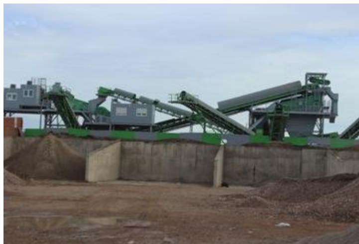
Figure II-17 Side view of the stationary plant
