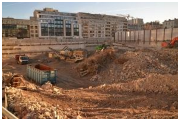
Figure II-51 Location of mobile crushing equipment on site
